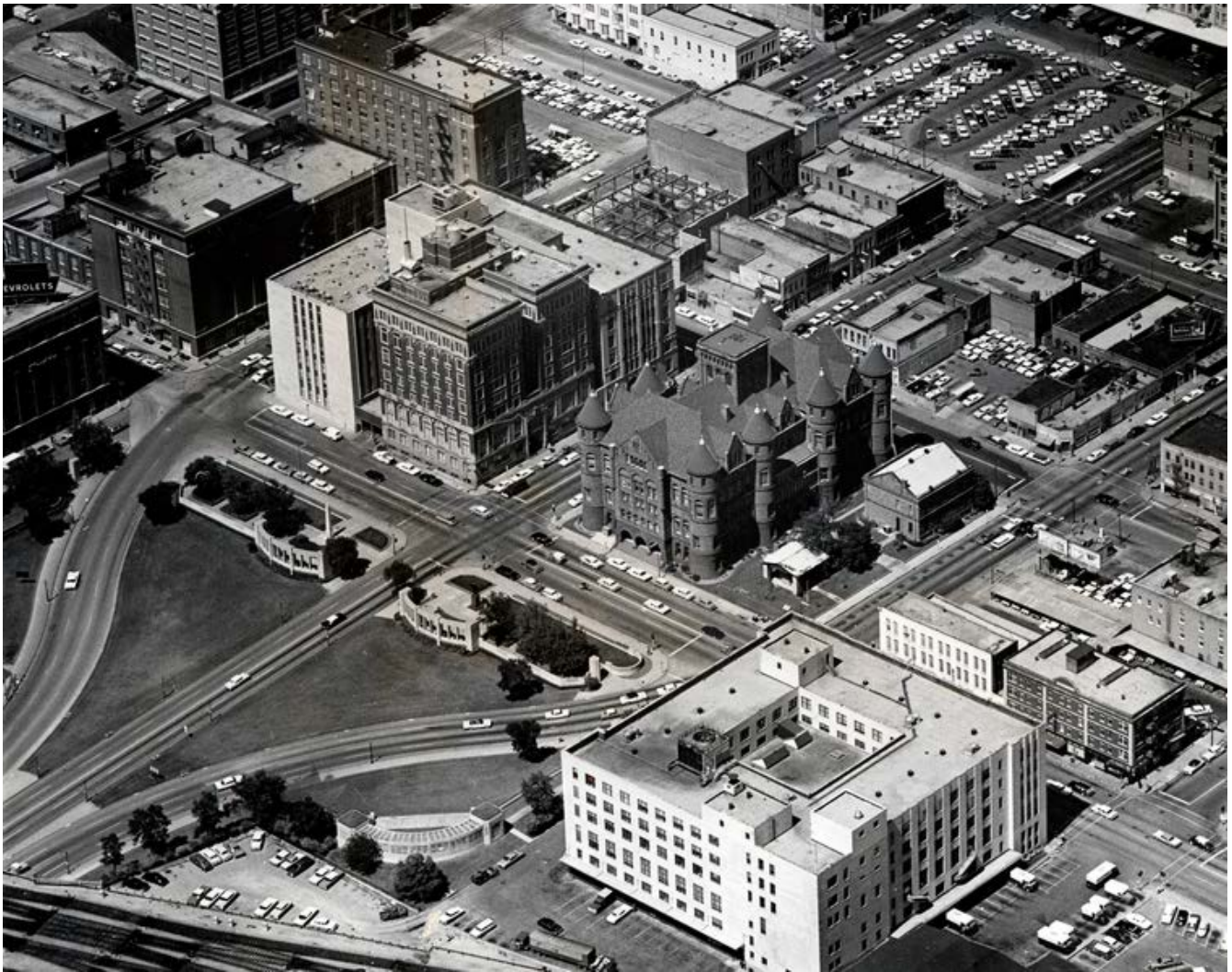
Left: The Triple Underpass under construction in 1935. The elegant moderne design, produced by highway department engineers, echoed the architecture of the contemporaneous Centennial Exposition at Fair Park. Right: An aerial view of Dealey Plaza and downtown Dallas in 1961. In this view, the area behind the turreted Old Red Courthouse has yet to be cleared to make way for Founder's Plaza and the JFK Memorial.
